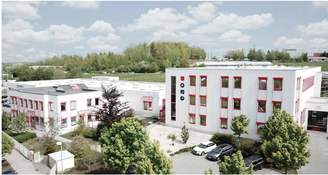
EAO Automotive HMI Centre of Excellence in Auerbach, Germany.
